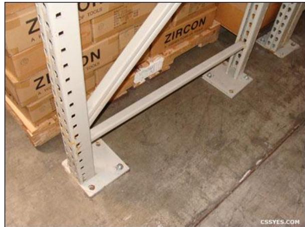
sprinklers. The IT infrastructure can be prevented from damage by using loop fasteners and hooks to servers, computers, network devices and other valuable items from falling. Also, installing anchors on pallet rack frames can secure your rack system to help avoid accidents during an earthquake event.
